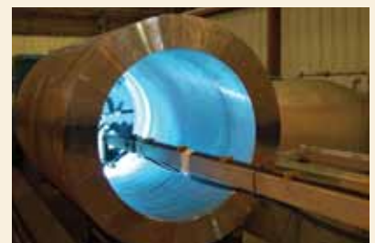
Bulkwelding process being applied to pipe
